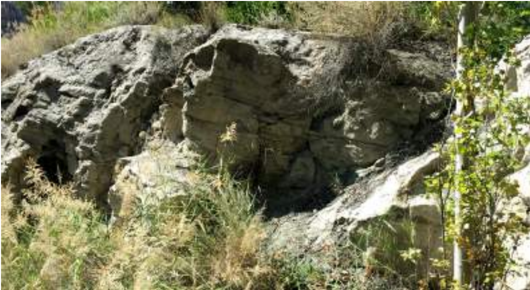
Photo 6-10 Tiltness in Clayey Silt Beds, Left Side of Road at Sarat Village.
