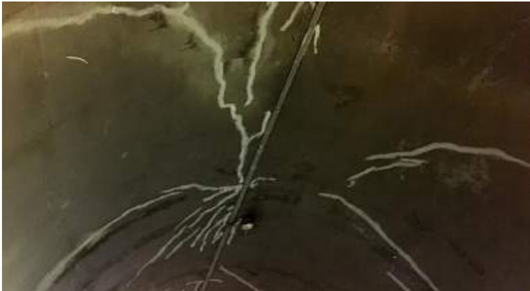
Photo 6-15 View of Recently Generated Joints Tunnel-2.
