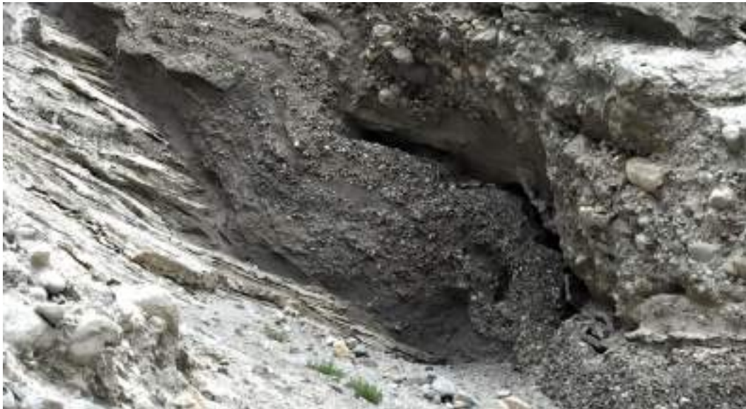
Photo 6-21 Inclination in Clay Silt and Gravels.
